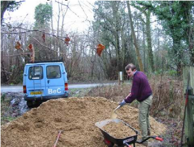
Neil with one of the first barrowloads of hogging.
