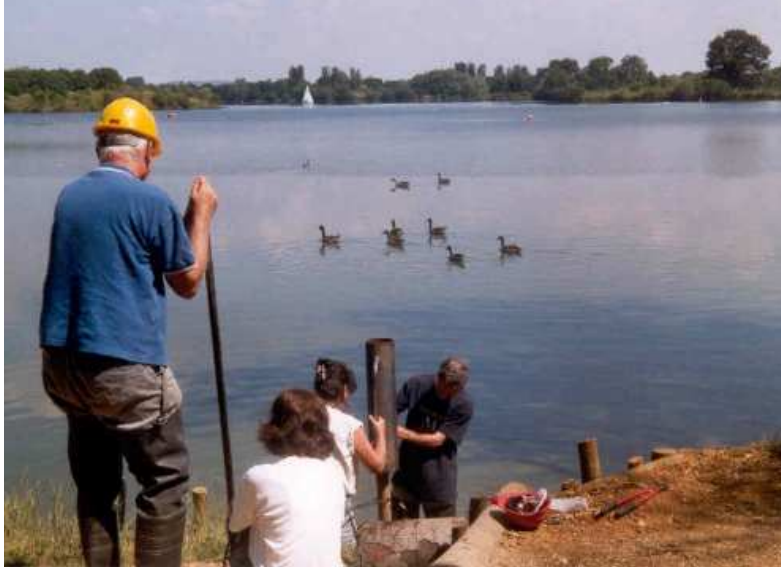
Knocking in posts to hold our log revetment in place in the lake at Dinton Pastures.
