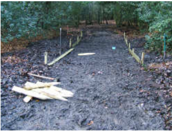
Above left - staking out the edging boards. Above right - putting down the brushings and gravel base layer. Below - Richard & Jon shovelling gravel into the Brava.
