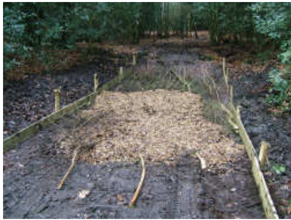
Above left - staking out the edging boards. Above right - putting down the brushings and gravel base layer. Below - Richard & Jon shovelling gravel into the Brava.
