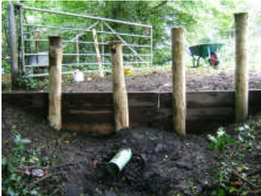
Above left – The almost finished revetment with the drainage culvert appearing at the bottom. The posts were trimmed later in the day. Above middle – the dismantled old bridge. Above right – the new bridge under construction, with everyone enjoying a well earned tea break in the background.
