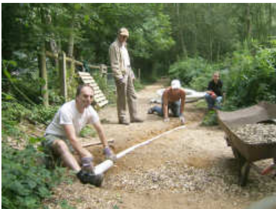
Above left – Phil, Peter, Richard & Aimee installing the drainage pipe across the path. Above right – the resurfaced section of path.
