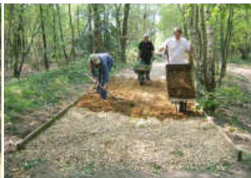
Above left – Peter & Nigel nailing the edging boards in place. Above middle - Jon & Nigel barrowing hogging whilst Sam spreads it out. Above right – the finished path.
