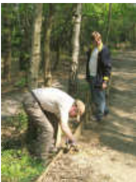
Above left – Peter & Nigel nailing the edging boards in place. Above middle - Jon & Nigel barrowing hogging whilst Sam spreads it out. Above right – the finished path.
