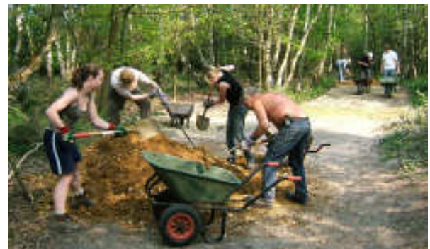
Right – Aimee, Peter, Amy & Richard shovel hogging into a barrow whilst Nigel, Jon & Sam deposit it on the path in the background.
