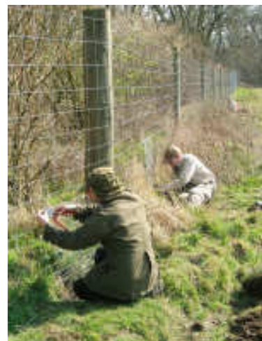
Phil & Peter working on the fence.
