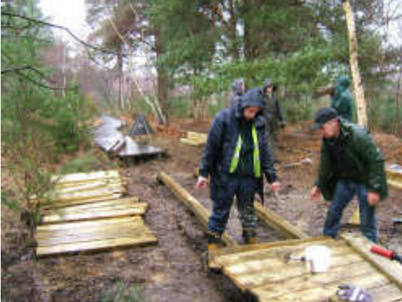
Above left Alisdair & Richard marking up the boards needed to get round a bend in the boardwalk. Above right – Peter, Owen, Richard & Gabriel look on as Alisdair cuts a board to size.
