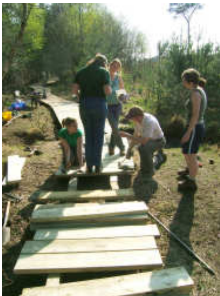
Above left – Fran & David dismantling a section of the old boardwalk. Above right – Amy nailing on the decking. Below left & middle – nailing on the new decking. Below right – the finished section of boardwalk.
