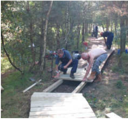
Left - Alisdair & Justin nailing the decking into place. Below left – Peter & Alisdair working on the bend. Below middle – Peacock butterfly. Below right – the finished boardwalk.
