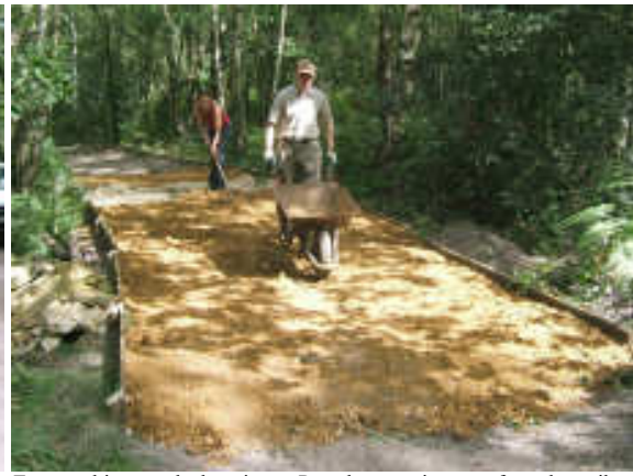
Above left – Peter, Richard and Vicky shovelling hogging Above right – Emma raking out the hogging as Peter barrows it across from the trailer
