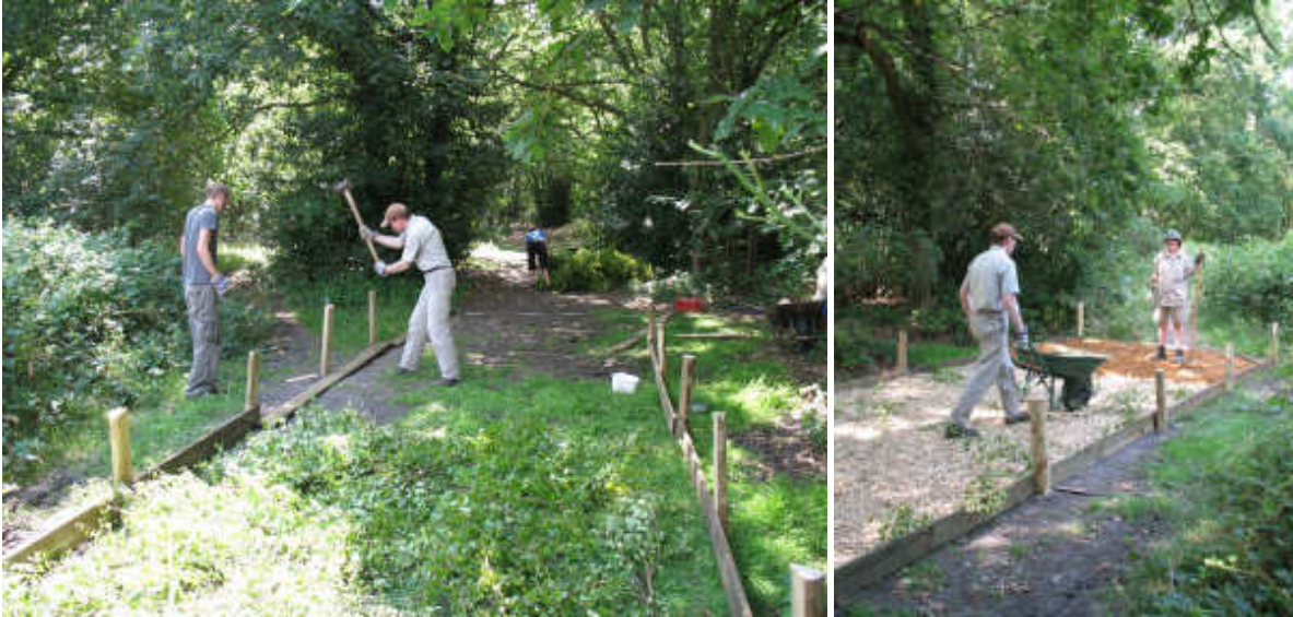
Above left – Dom & Peter knocking in stakes. Above right – Peter and Vicky spreading hogging . Below left – Dom & Gemma barrowing hogging. Below middle – Gemma raking out the gravel. Below right – the finished path.
