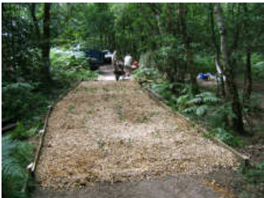
Left – the gravel layer in place.
