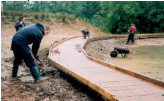
Alisdair shovelling mud!
