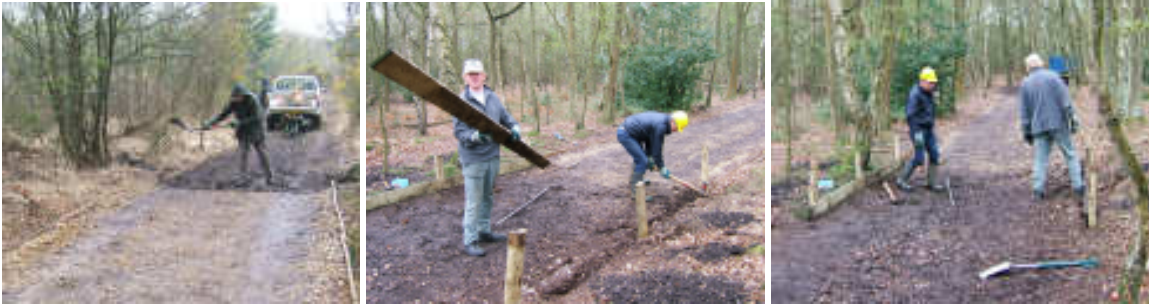
How to resurface a bridleway – 1) Peter clearing some of the mud. 2&3) Mark & Richard installing the edging boards. 4) Add a layer of brashings, followed by gravel 5) Peter & Nigel barrowing gravel. 6) Richard & David trimming off the posts.
