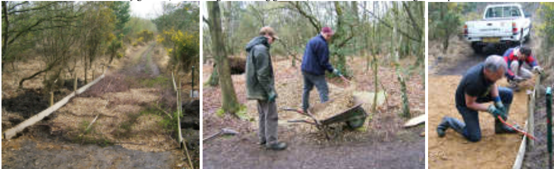
How to resurface a bridleway – 1) Peter clearing some of the mud. 2&3) Mark & Richard installing the edging boards. 4) Add a layer of brashings, followed by gravel 5) Peter & Nigel barrowing gravel. 6) Richard & David trimming off the posts.
